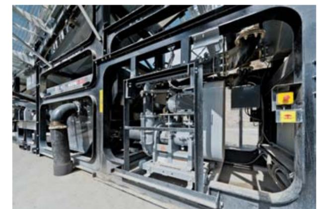
Centrifugal Pumps, Roll out for Service Access
