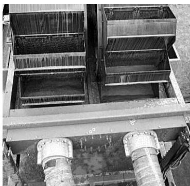
Anti-turbulence inlets in bucket tank
