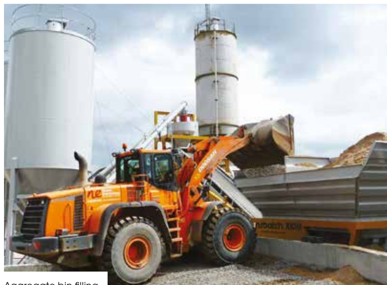
Aggregate bin filling
