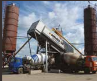
Concrete road building and readymix Russia
