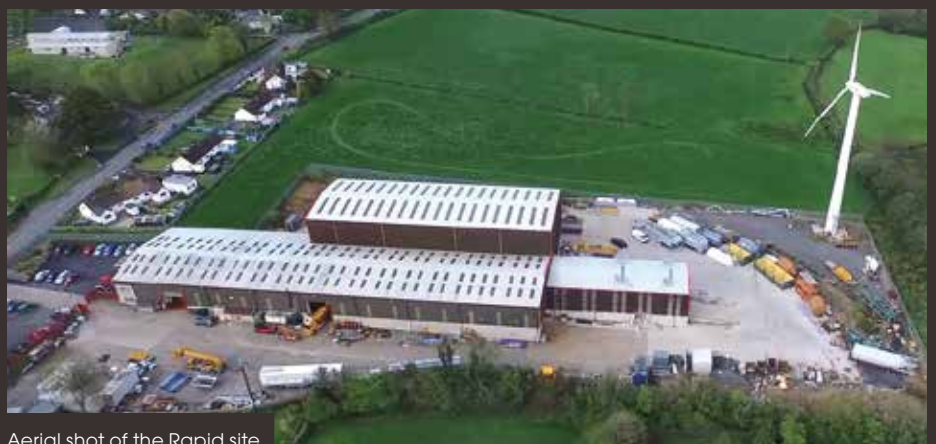
Aerial shot of the Rapid site
