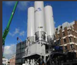
Rail Project England
