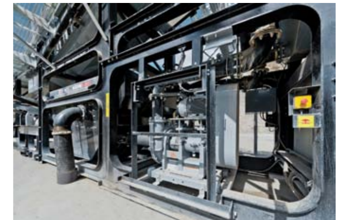
Centrifugal Pumps, Roll out for Service Access
